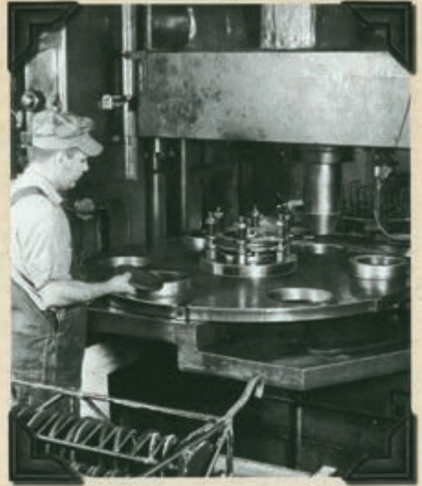
A Summer 1953 Knuckle Joint Press for 105 mm cartridge cases for howitzers
